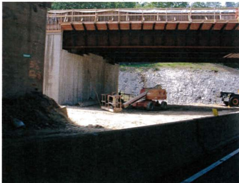
Figure 2. Society Road Bridge over I-95 in East Lyme at Exit 73 (Photograph by Greg Stroud, June 4, 2016).
